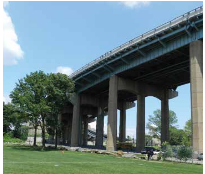
Figure 4. Ward's Island viaduct structure. Courtesy of Thornton Tomasetti Weidlinger.
