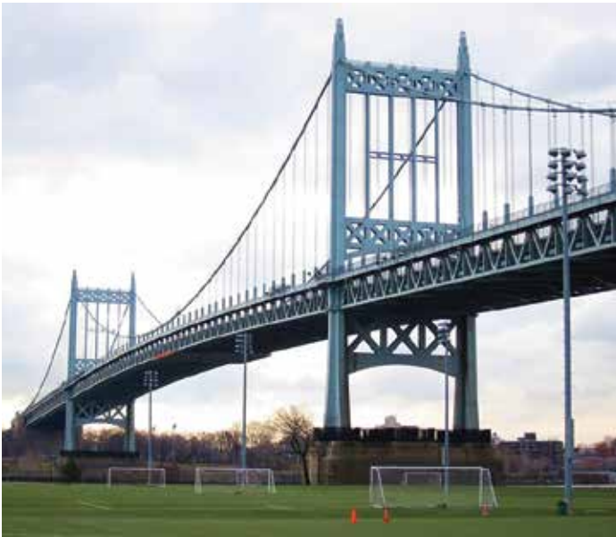
Figure 2. Suspended span. Courtesy of Thornton Tomasetti Weidlinger.
