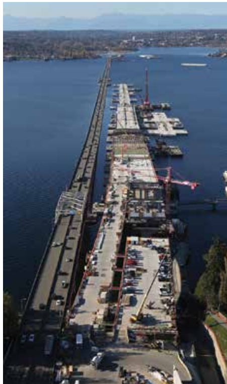
Aerial view of mainline bridge and BCD raft pontoon.
