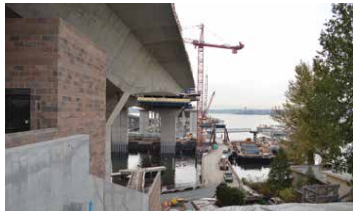
Land to water access trestle.
