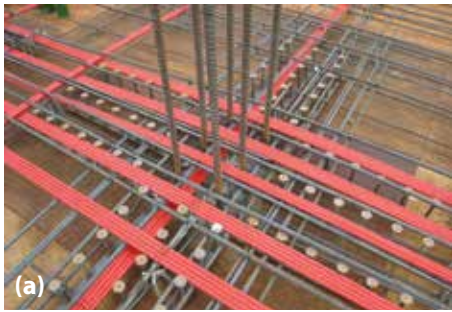
Figure 2. Two-way slab construction with unbonded and bonded post-tensioning tendons. (a) Slab construction with unbonded tendons. Neither ACI nor EC2 requires a strength check at the initiation of cracking (P998). (b) Slab construction with bonded tendons ACI requires a strength check at the initiation of cracking. EC2 does not (P999).
