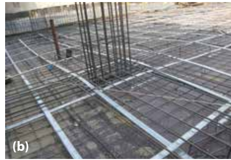
Figure 2. Two-way slab construction with unbonded and bonded post-tensioning tendons. (a) Slab construction with unbonded tendons. Neither ACI nor EC2 requires a strength check at the initiation of cracking (P998). (b) Slab construction with bonded tendons ACI requires a strength check at the initiation of cracking. EC2 does not (P999).
