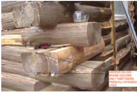
Figure 4. Log profile; note reveal for the spline.
