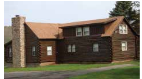
Figure 7. Log cabin after wall repair.
