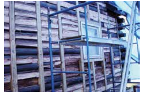
Figure 6. Staging of repair in progress.
