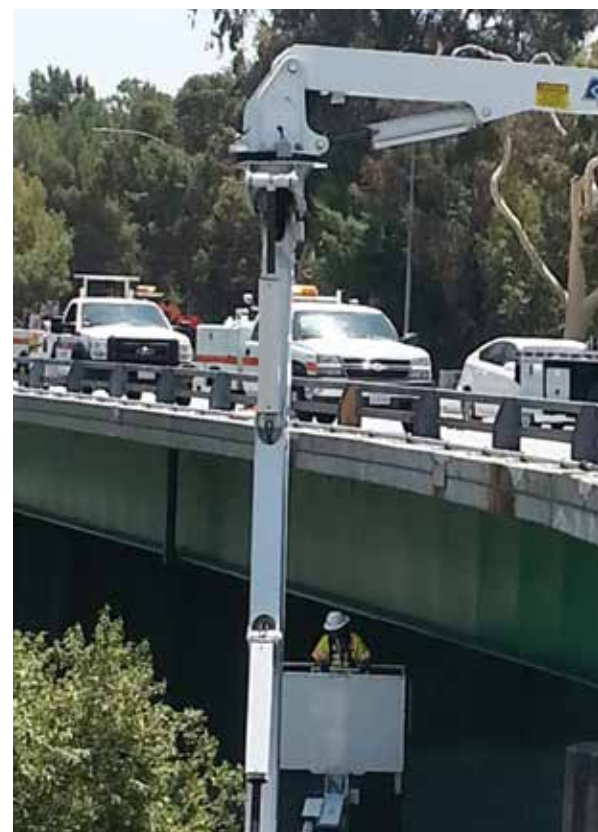
Figure 2. Under bridge inspection truck (UBIT).
