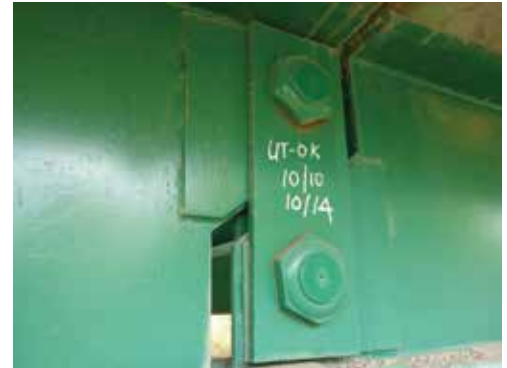
Figure 1. Pin-and-hanger assembly.
