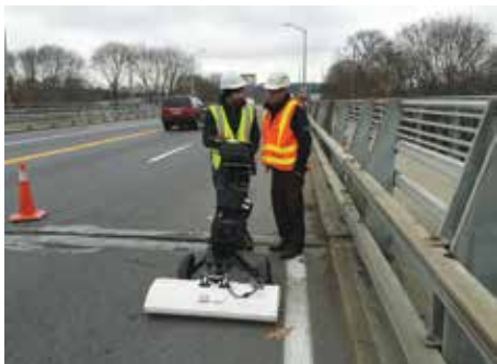
Figure 6. Multi-array Bridge Inspection Unit in operation scanning bridge deck arrangement and condition. Courtesy of Echem Consultants LLC.
