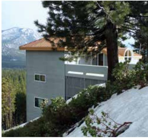
Figure 1. Typical hillside house with upper level garage.
