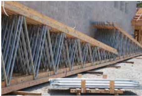
Figure 6. Delivered segments before assembly. Once assembled, they will form a 75-foot-long scissor pitched truss. Note the required steel-tube cross-bracing in the foreground.
