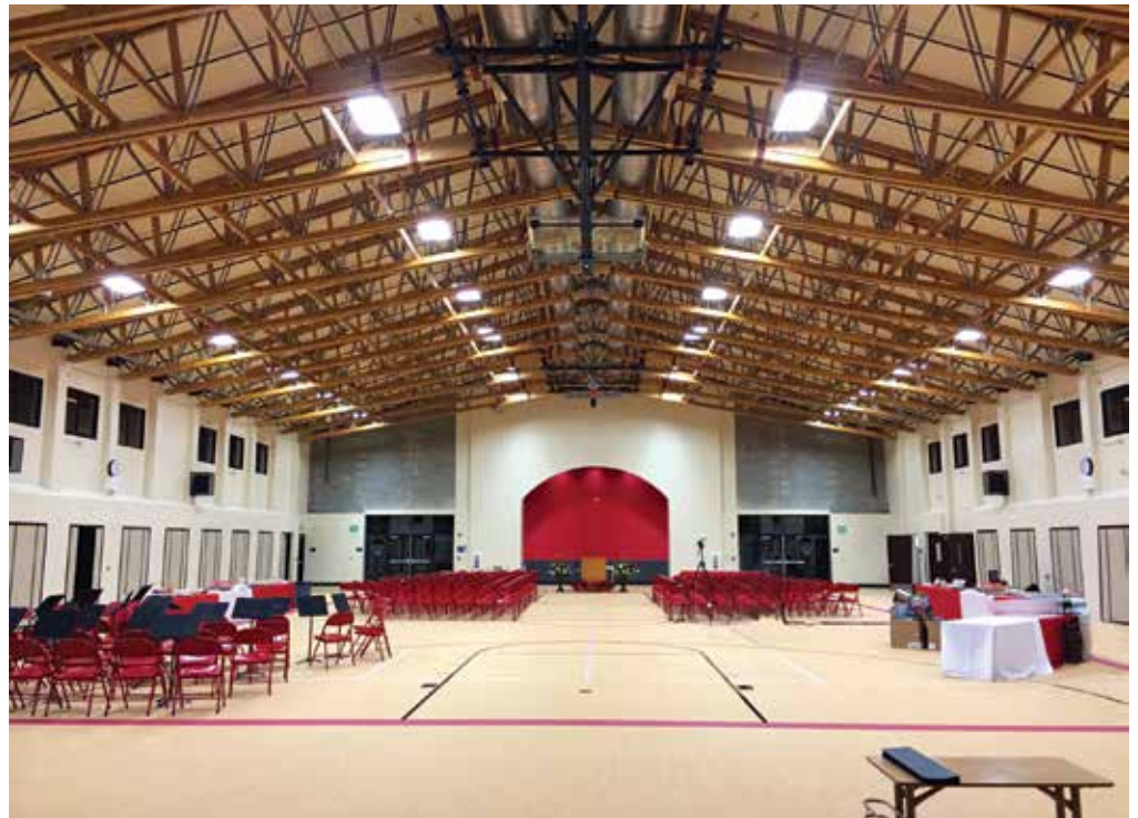
Figure 1. Exposed trusses create visual appeal for the Taylor Middle School cafeteria and public meeting space.
