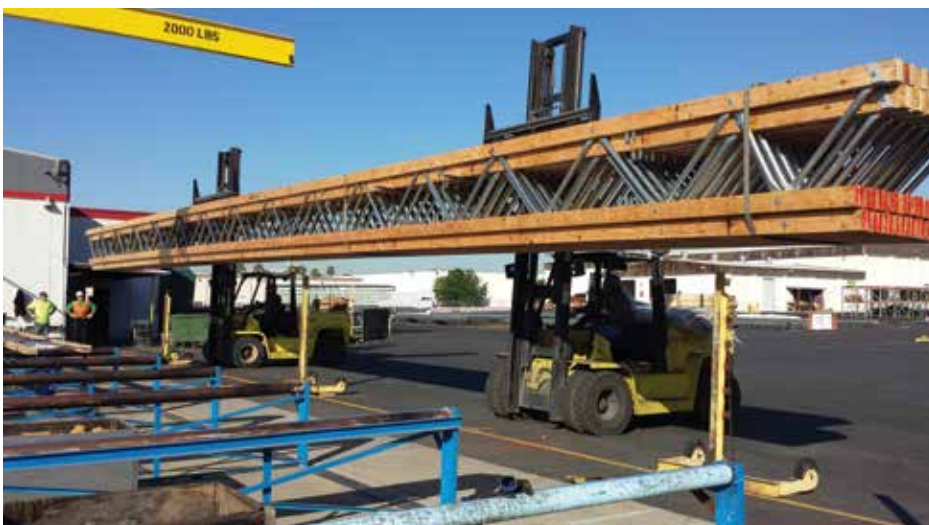
Figure 4. Proper forklift spacing and fork locations ensure trusses are not damaged during handling.
