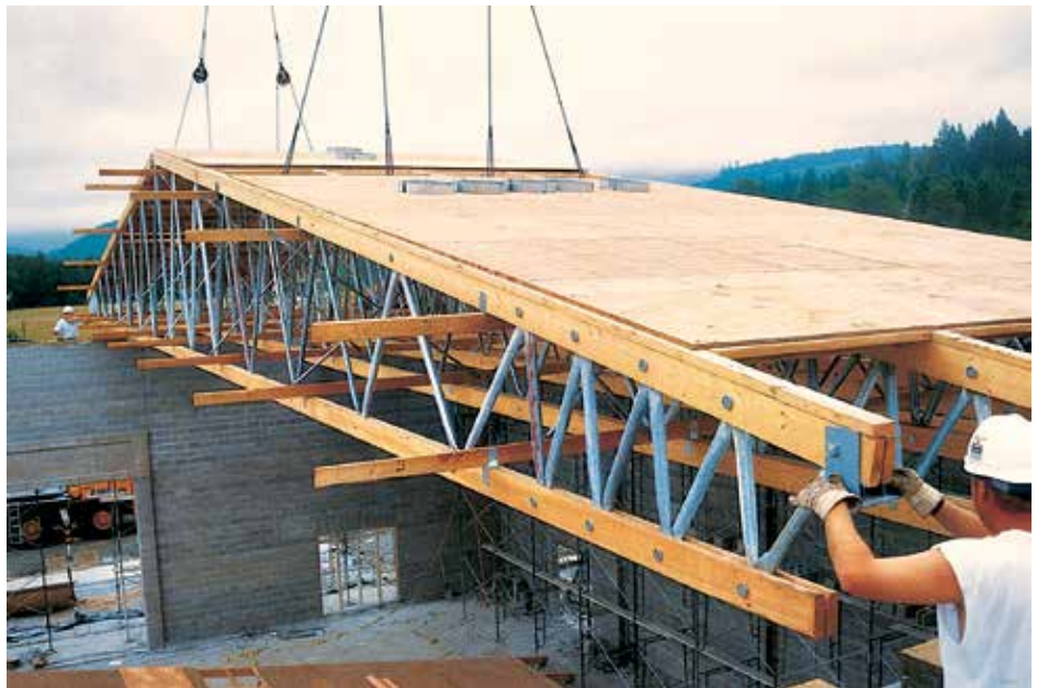
Figure 3. Workers are guiding a module of pitched trusses into place.
