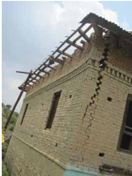
Figure 8. Out-of-plane failure of exterior adobe walls.
