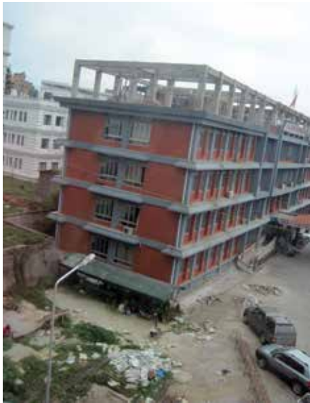
Figure 5. Brick in cement mortar infill in RC frame systems in Kathmandu.
