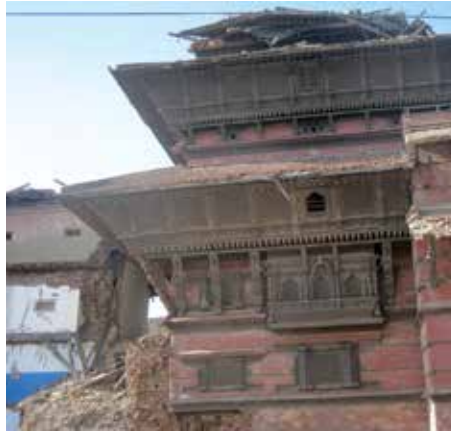
Figure 7. URM wall failure of the Kathmandu Durbar square.
