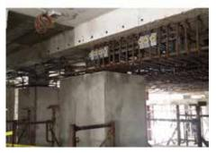
numerous eccentric pile caps to keep all new piles at the tower perimeter inside the garage footprint, allowing occupancy of the retail shops to remain undisturbed. Since access to the FP&L electric room was forbidden, MC designed a 2-story tall 60-foot long post-tensioned beam to transfer the overstress portion of the column and foundation in the electric room to the adjacent building columns which were strengthened for the additional load.
