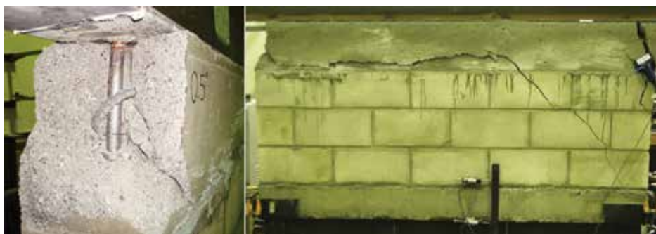
Figure 9. Breakout failure of test specimen with 4 headed studs.
