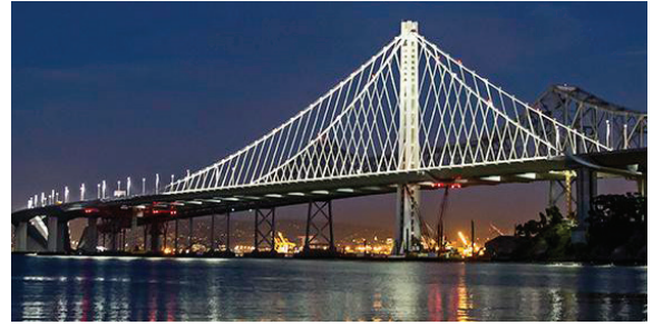
Self-anchored suspension (SAS) on the main span of the East Span of Bay Bridge.
