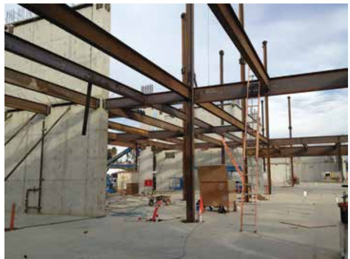
Steel framing and concrete shear walls.
