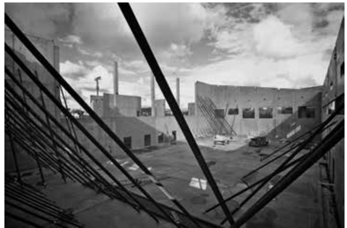
Erected tilt-up panels.
