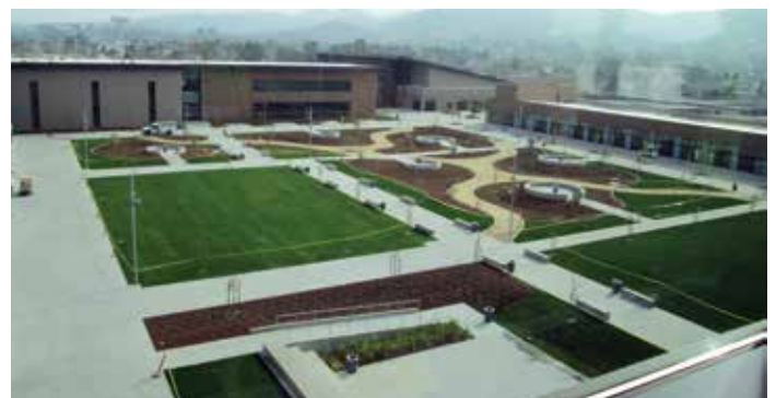
Art, gymnasium and shop buildings and central quad area.
