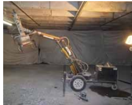
Figure 3. Remotely operated excavation hammer.
