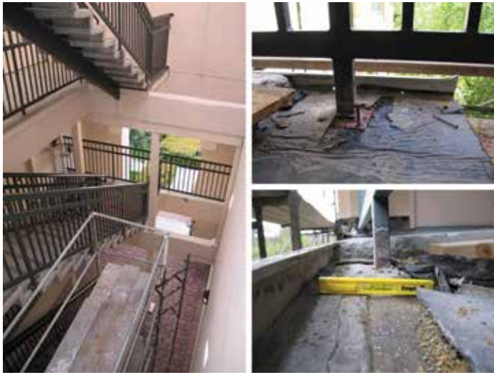
Figure 3. Detail creates a reverse slope.
