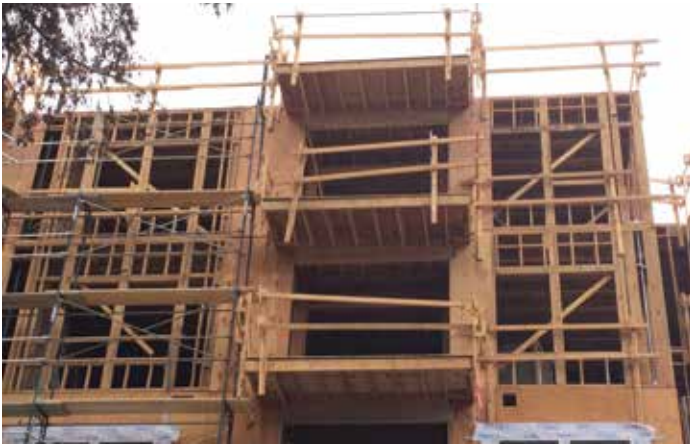
Figure 1. Common wood balcony configuration under construction.
