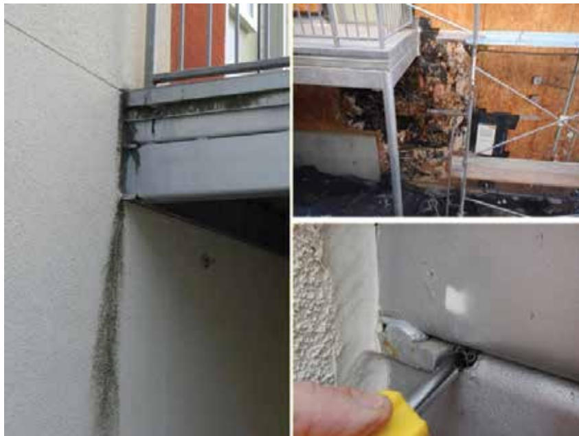
Figure 9. Steel stair landing. Images are actually taken from multiple examples of this landing type.
