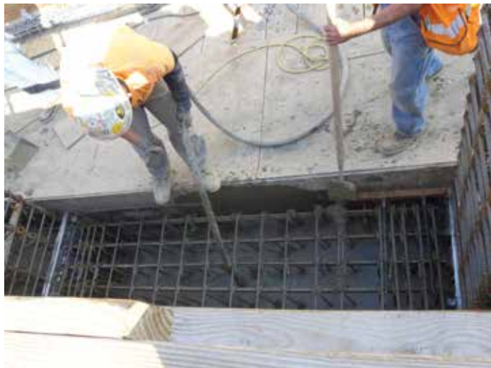
Steel fiber reinforced concrete shear wall coupling beam under construction.
