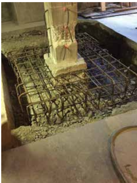
Figure 4. Footing extension reinforcing at existing caisson foundation.
