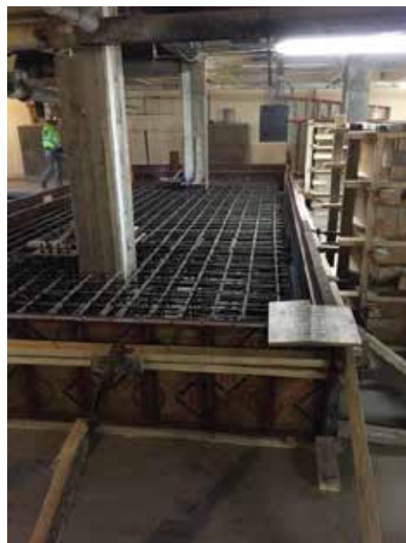
Figure 5. Braced frame uplift resisting mat footing.
