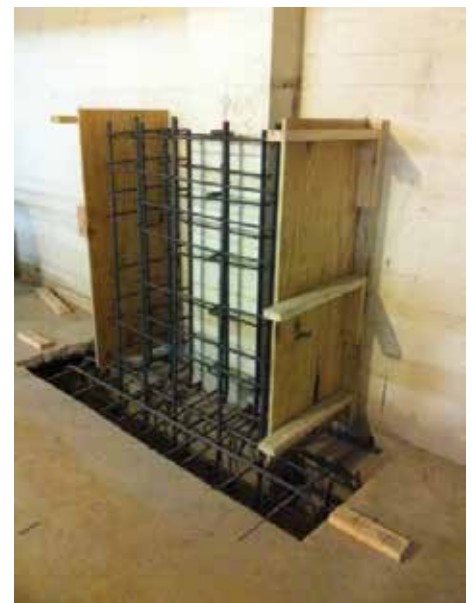
Figure 6. Existing column concrete collar reinforcing.
