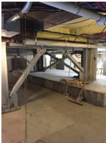
Figure 2. Center core braced frame at basement level.
