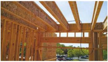
*I-joists bearing at an exterior wall and a laminated veneer lumber header over a window opening.*
