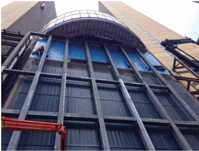
Figure 3. Vierendeel truss.
