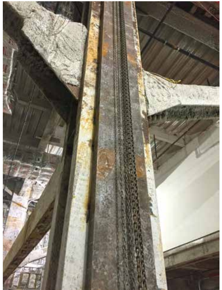
Figure 6. Column reinforcing.
