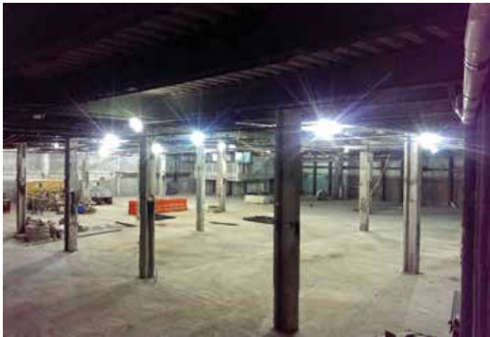
Figure 5. New double story space with reinforced columns.
