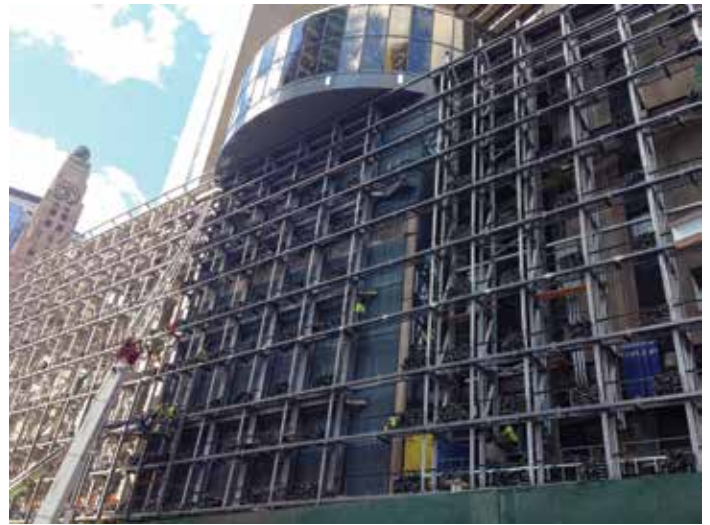
Figure 4. Installation of LED sign.
