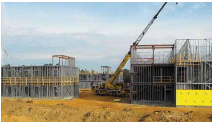
Figure 1. 3-story cold-formed steel framed multi-family residential building.
