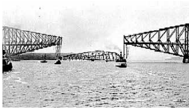
Suspended span collapsing into the St. Lawrence River.
