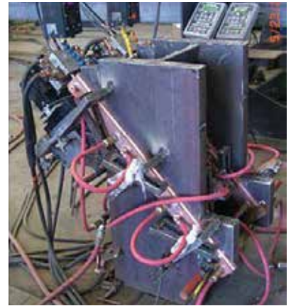
Mock-up of instrumented column flange splice. Traditional horizontal FCAW column splices can be rapidly welded at 45 degrees using ESW-NG.
