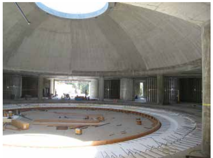
Figure 2. Main dome over Prayer Hall during construction.
