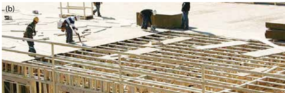
Figures 3a and 3b. Periodic special inspection is required for nailing, bolting, anchoring and other fastening of elements of the seismic and main wind force-resisting systems, including wood shear walls, wood diaphragms, drag struts, braces and hold-downs.
