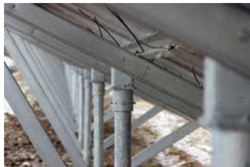
Hot-dip galvanizing protects the buried steel supports of the Discovery Light Solar Project in Beaverton, Ontario, Canada.
