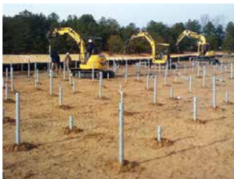
Magnum Piering, Inc.'s helical pilings in Westchester, Ohio rely on hot-dip galvanizing for corrosion protection.
