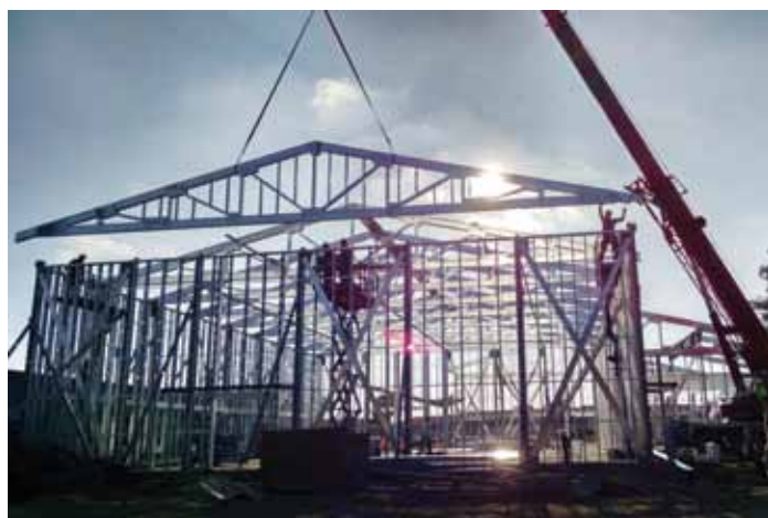
Figure 3. Gable end trusses keep the wall stud depths to a minimum. Courtesy of Yaroslav Derdyk, Broward Builders, Inc.
