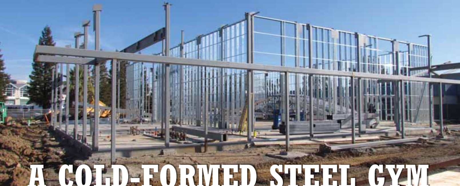
Figure 1. A regular grid of HSS columns surround the main gym and auxiliary spaces.
