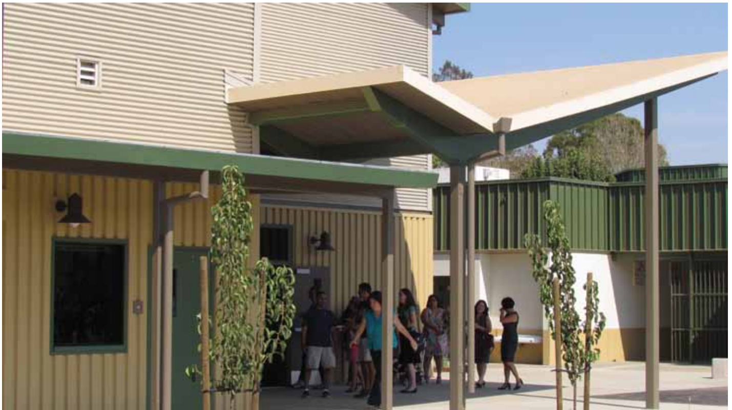
Figure 4. Profiled steel panels provide an attractive and economical exterior finish.
