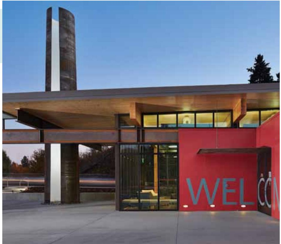
up in place. To control cracking and provide durability, the letters were reinforced with a welded rebar mesh. KPFF designed the lifting brackets and erection assemblies to support the letters and minimize stresses while they were being erected.
