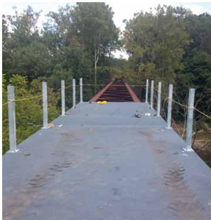
Figure 6. FiberSPAN panels fastened to the top of the bridge's steel superstructure.
