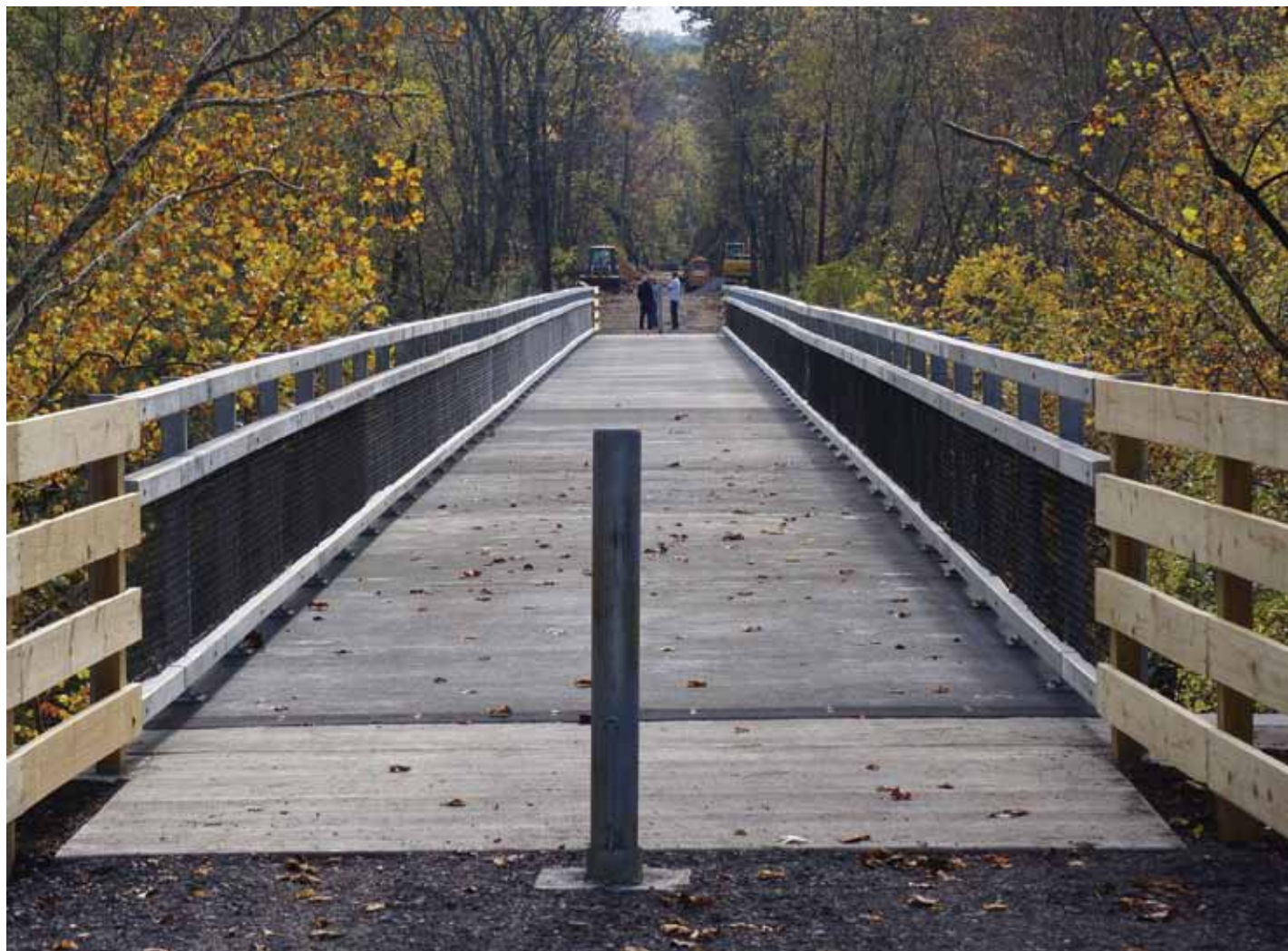
Figure 7. Blending with its natural surroundings, the FRP bridge deck gives pedestrians safe passage across the river and access to new trail sections.
