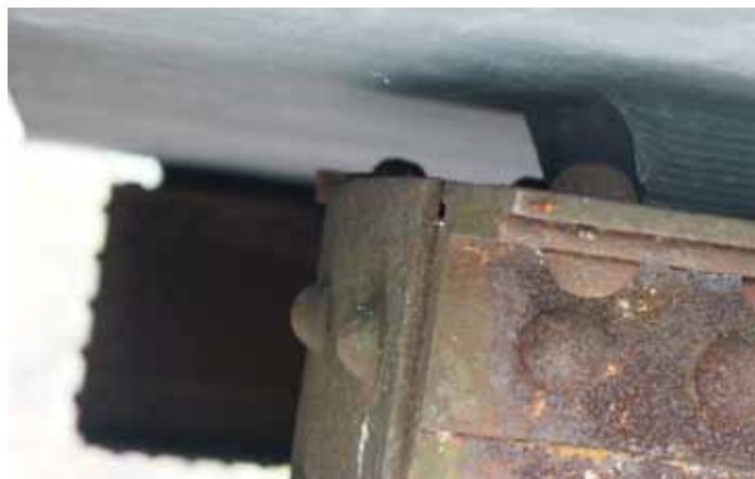
Figure 2. The integrally molded step secures the deck panel to the steel superstructure without the need for secondary shim pieces.
