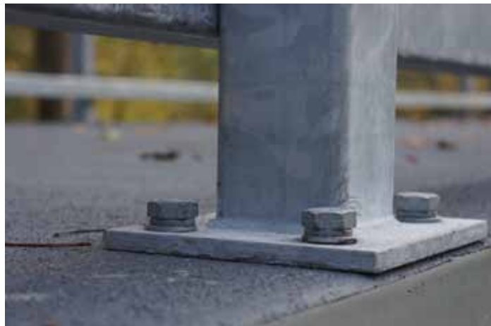
Figure 3. FRP is robust enough to handle rail post attachment load.
