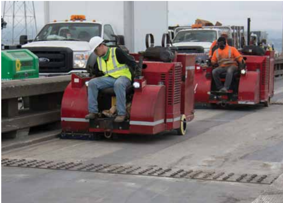
Figure 2. Deck being shotblasted after removal of old EAC. Note: Transverse bolted splice plate in foreground.
