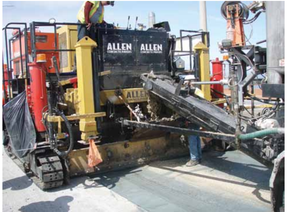
Figure 3. Continuous mixer/batching truck discharging into paver. Prepared surface has a coating of the methacrylate prime coat containing 85% by weight zinc powder as a corrosion inhibitor.
