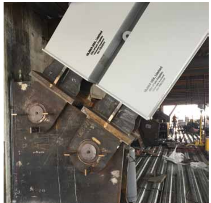
Figure 6. Gusset plates and BRBs installed.
