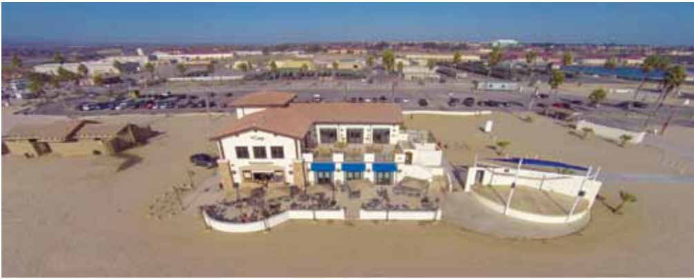
Figure 1. Completed multi-use facility.
