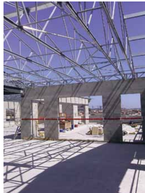
Figure 4. CFS roof trusses employed at the multi-use facility.
