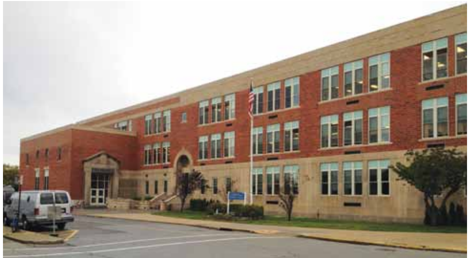
Figure 6. Completed system on steel frame buildings.
