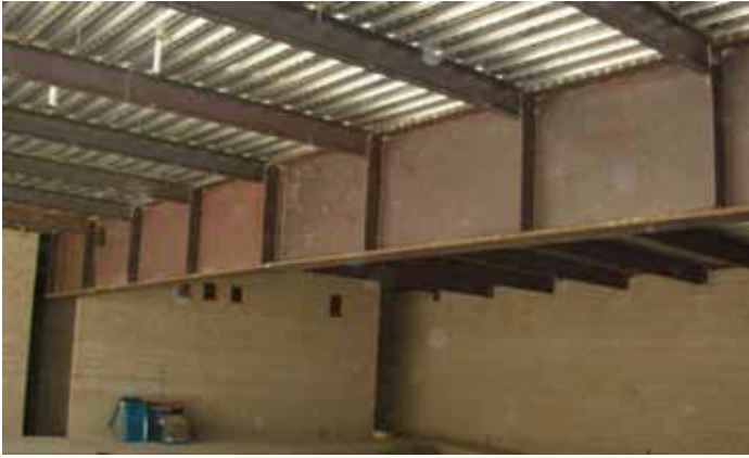
Figure 3a. Construction photo inset of 5-foot deep tapered steel girder.
