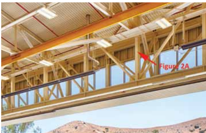
Figure 2a. Box truss.
