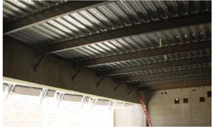
Figure 3b. Construction photo inset of 8-foot deep concrete transfer girder.
