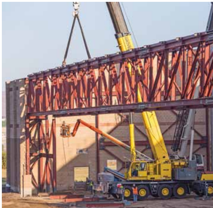
Figure 4. Field-fabricated truss for hangar.
