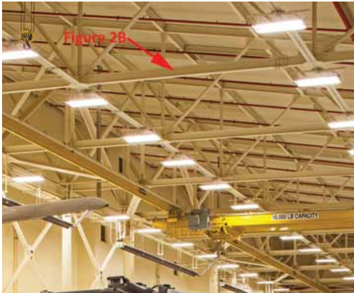
Figure 2b. Transverse truss.
