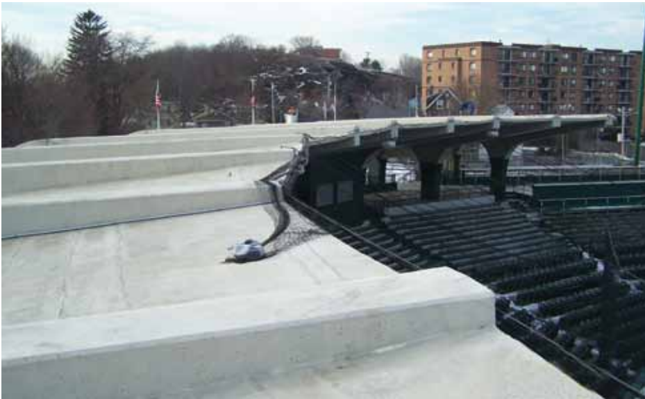
Upturned beams at a stadium.
