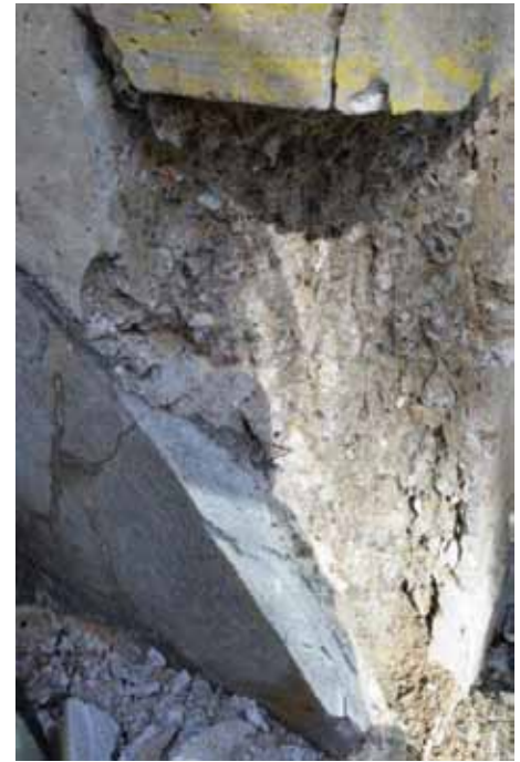
ASR deterioration.
