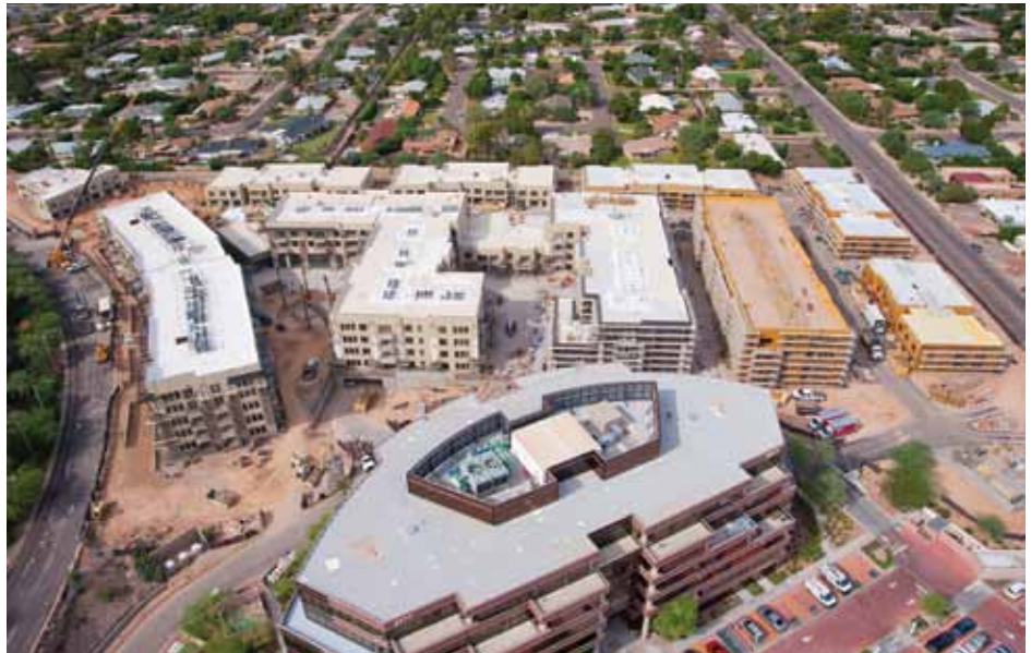
A coalition of stakeholder organizations involved in the construction of large buildings has joined together to develop education and training materials on how to reduce the frequency and severity of fires during construction.
