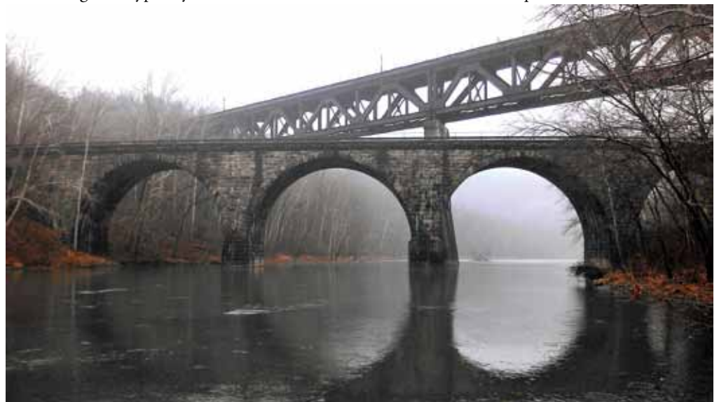
Six-span, railroad stone arch bridge constructed in 1907 over Conemaugh River, Pennsylvania. It was later replaced by a new steel truss bridge when the railroad was realigned due to construction of the Conemaugh River Dam.
