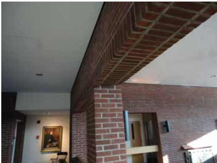
Figure 4. Interior openings with masonry beams.
