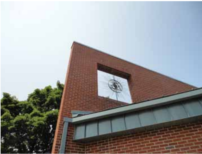
Figure 10. Aesthetic brick beam.
