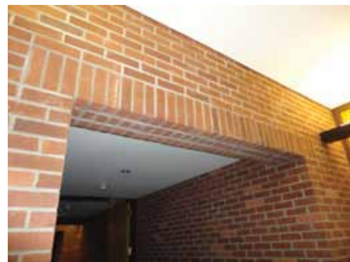
Figure 2. Interior brick beam.
