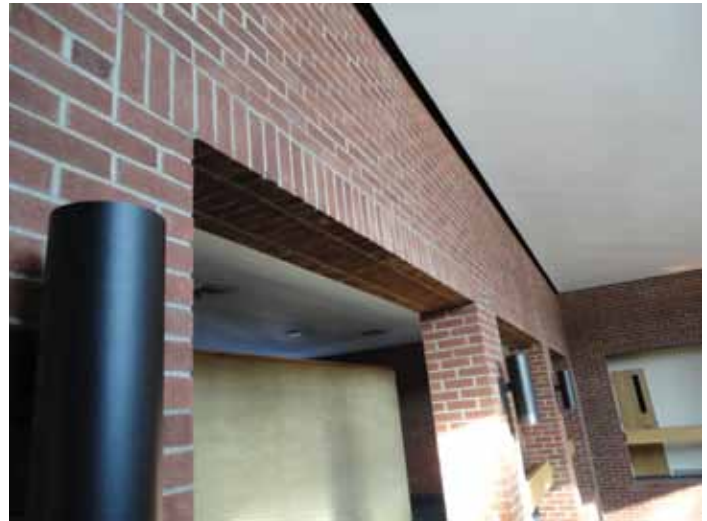
Figure 5. Interior openings with steel framing.
