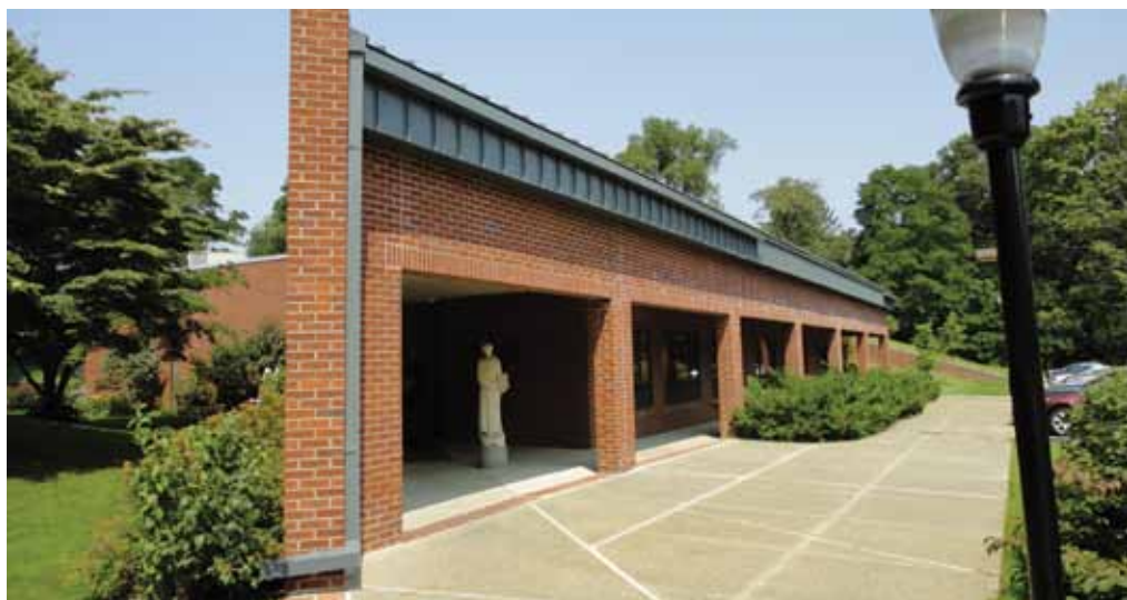
Figure 1. East entrance into common area (2014).
