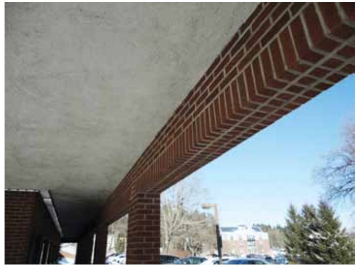
Figure 11. Brick beams at entry.
