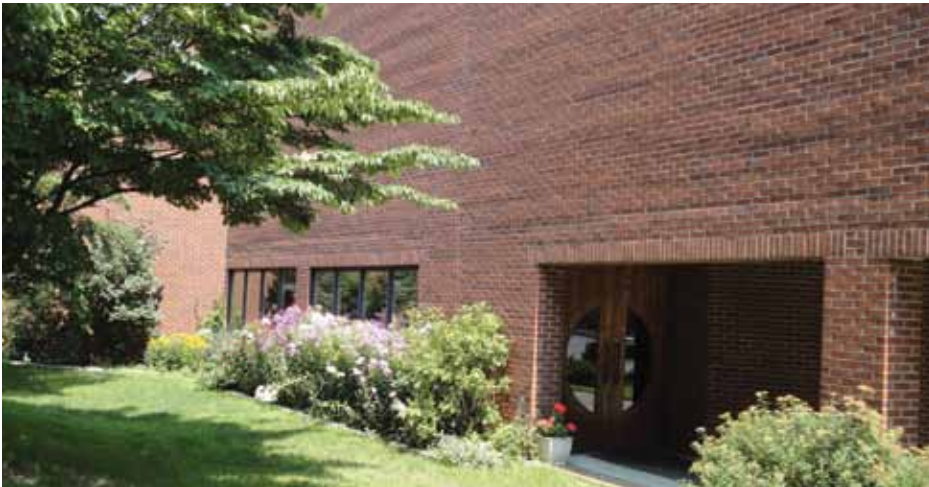
Figure 7. Exterior brick beams.
