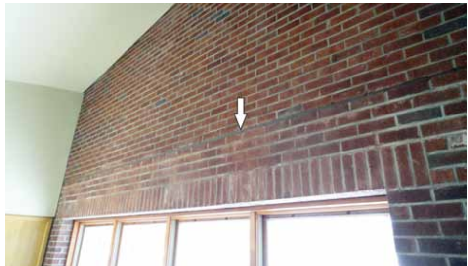
Figure 9. Interior of exterior wall beam.
