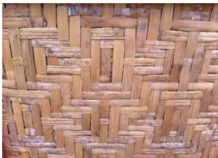
Figure 2. Amakan fabric used for siding.
