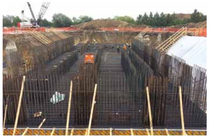
Figure 3. Concrete mat foundation.
