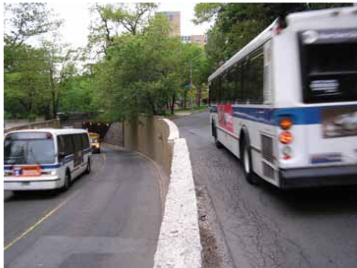
Figure 3. Leaning segment of retaining wall.
