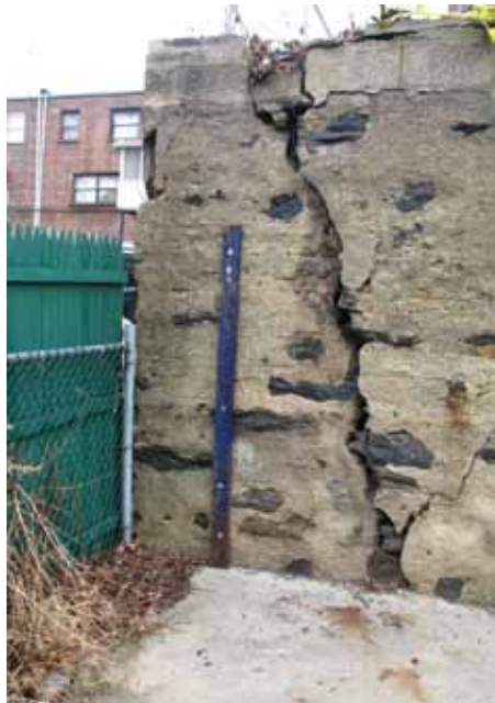
Figure 4. Severe crack in stone retaining wall.
