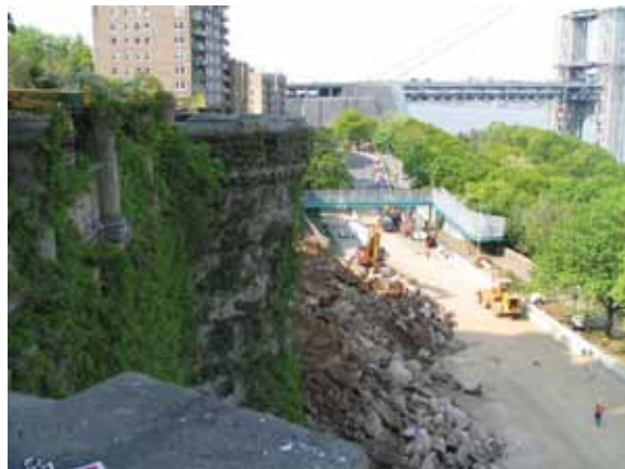
Figure 1. Collapsed retaining wall at Castle Village.
