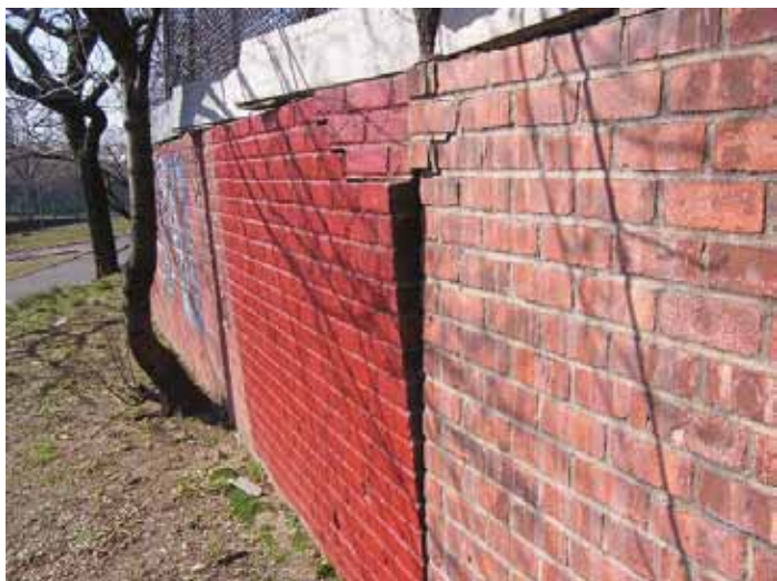
Figure 2. Cracked and leaning retaining wall brick veneer.
