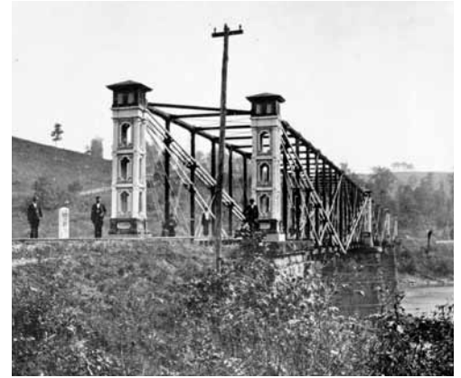
Monongahela Bridge 1865 – 1887, note skew. Courtesy of HAER.
