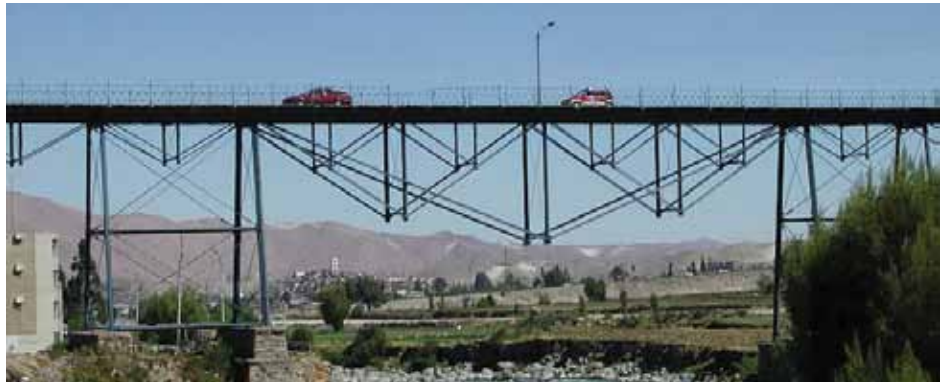
Rio Chili Bridge. Courtesy of Mark Yashinsky.
