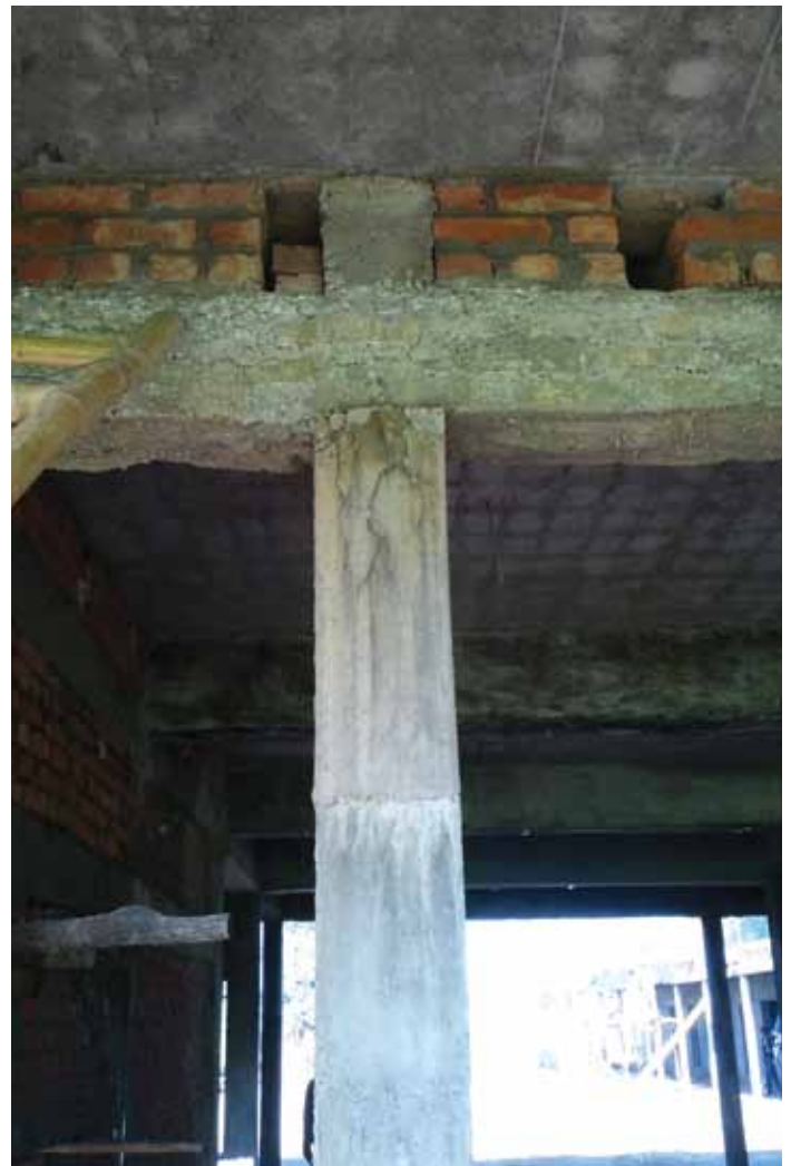
Roof slab supported by column and bricks.
