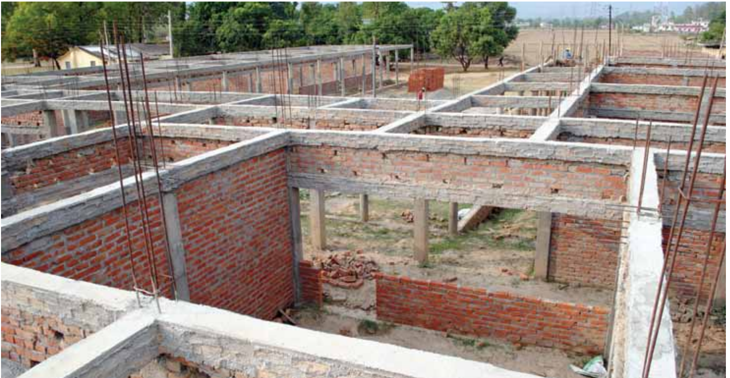
Roof beams poured independently from the slab.
