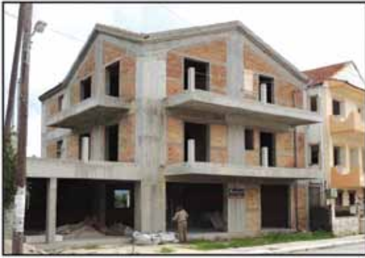
Figure 4. Typical confined masonry construction in Greece, with the infill masonry having concrete beams around openings, dowelled into the concrete structure (left). Characteristics of typical hollow clay bricks used for infill (right), after Xalkis Bricks (2015).
