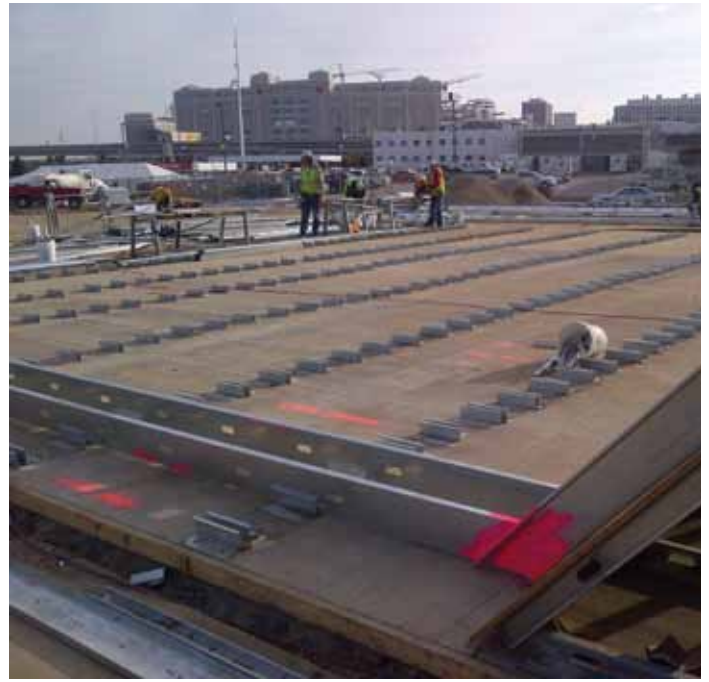
Figure 6. "Jig Table" used for on-site panel construction.
