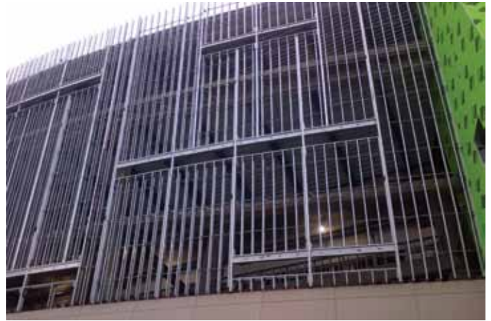
Figure 3. Staggered stick-framed openings at the west building elevation.
