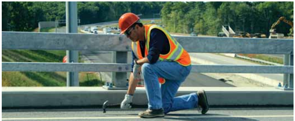
Figure 1. NDT testing procedure, called hammer sounding, using an acoustical representation to identify areas of delamination.
