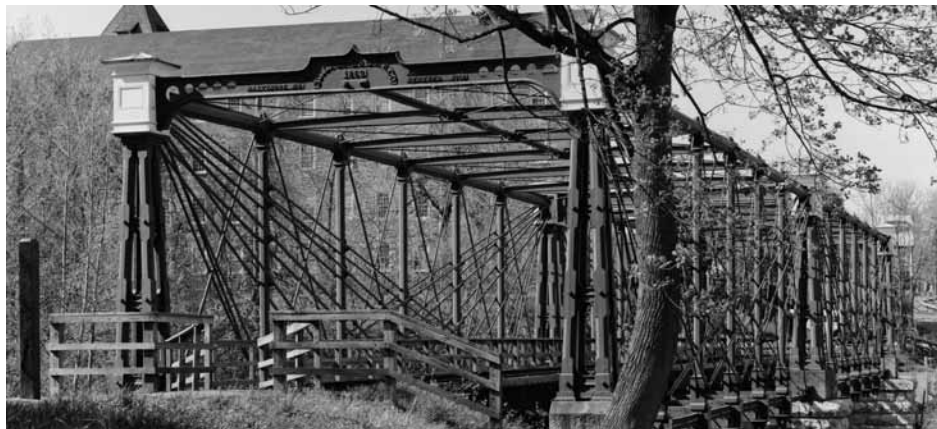
Bollman Bridge, Savage, Maryland. Courtesy of HAER.
