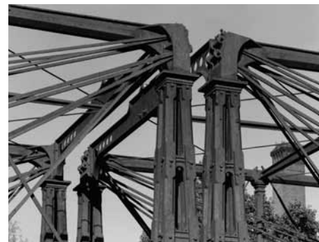
Bollman Truss, cast iron columns and top chord, wrought iron diagonals. Courtesy of HAER.
