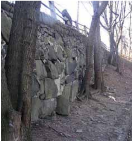
Figure 4. Bulging wall.
