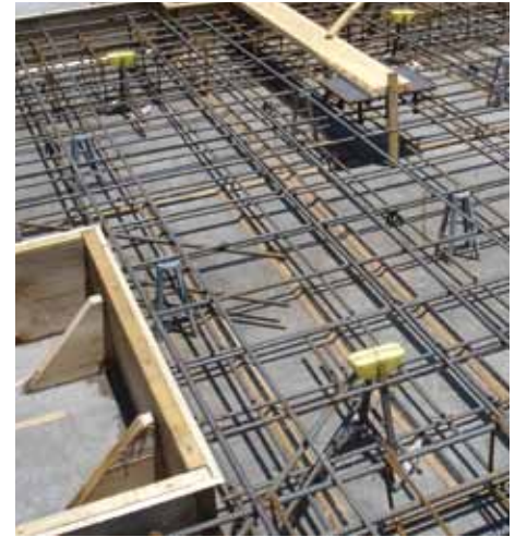
Figure 6. Diagonal corner bars to control cracking.
