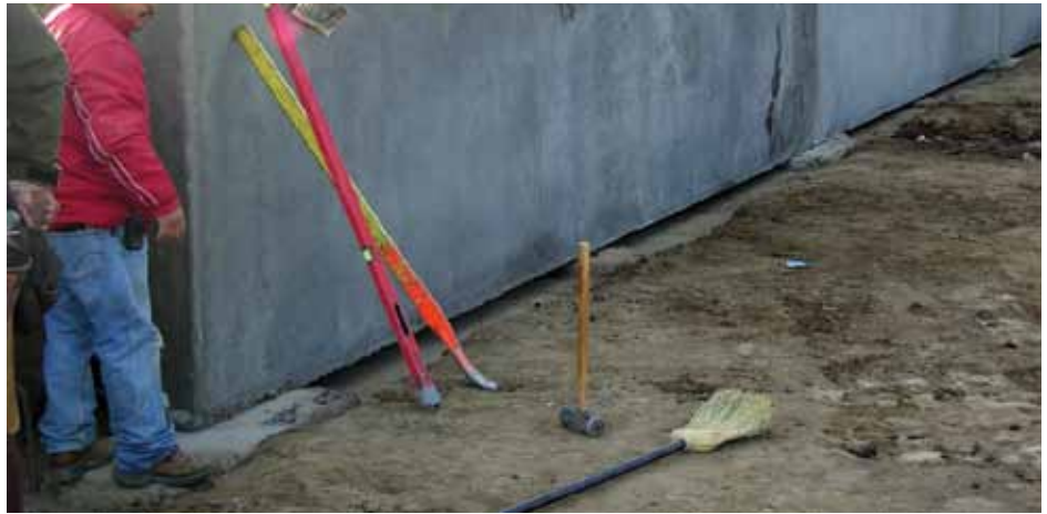
Figure 2. Grout setting pads at panel joints with an inactive shim at the panel center.
