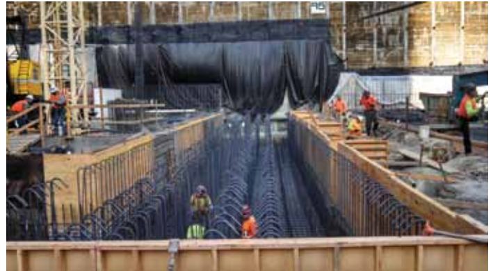
Grade beam with one million pounds of reinforcing.
