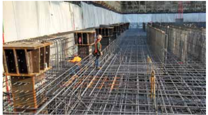
Mat reinforcing with shear reinforcing.
