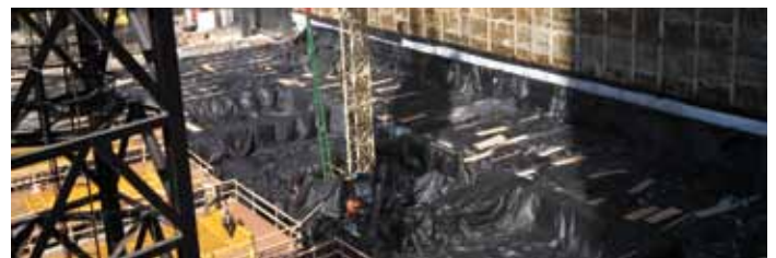
Insulating the mat for two weeks to keep extremities warm.
