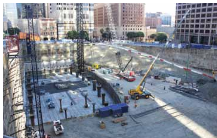
Rat slab with starter columns.
