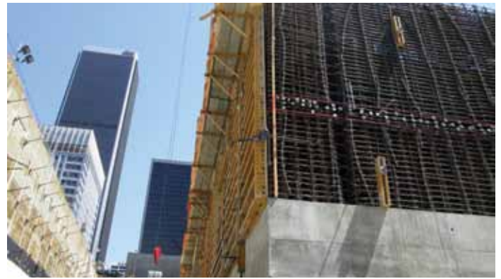
Typical corewall reinforcing.
