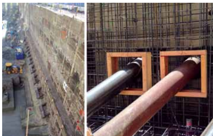
Shoring along 7 th street.
