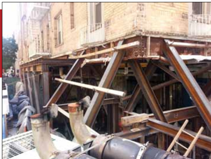
Figure 1. Elevation of temporary shoring system at north storefront and bearing wall.
