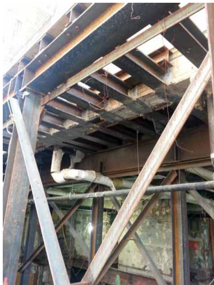
Figure 6. Needle beam support at existing masonry bearing wall with window distribution beam.
