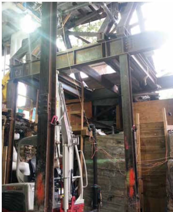
Figure 3. Elevation of northwest corner with post-tensioned pier supporting the A-Frames.
