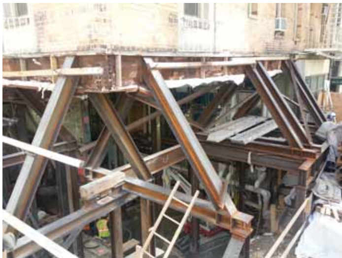
Figure 2. Typical A-Frame shoring at storefronts.
